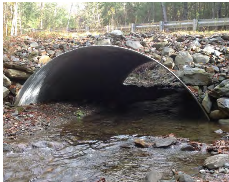
This culvert/bridge beneath Hale Road allows good passage for mammals and aquatic organisms.
