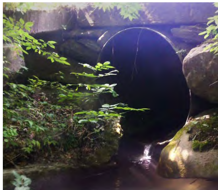
A hanging culvert under Old Stage Road is a barrier to aquatic organism movement.
